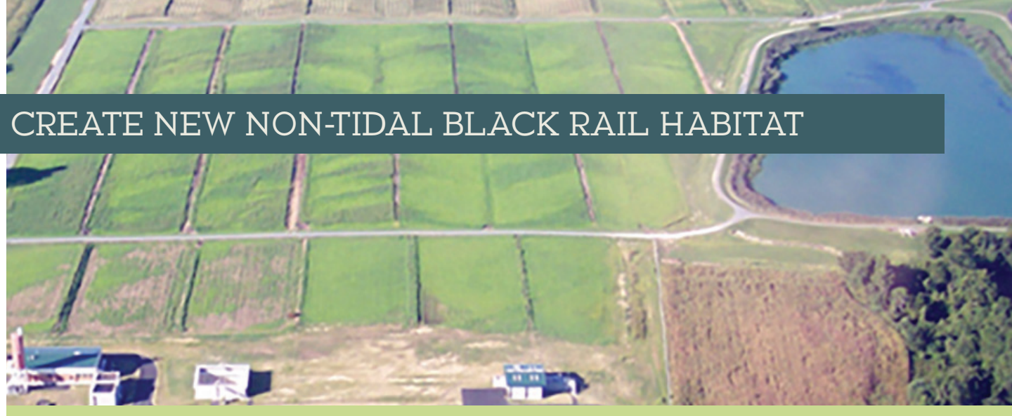
Inland non-tidal sites such as the Easton Water Treatment Plant holds promise for providing future habitat for Black Rails. Easton Water Treatment Plant
