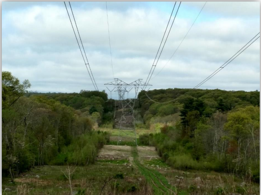
A utility right-of-way span managed for Golden-winged Warblers. Only 1/3 of the span is cut every 3 years. In 2019 the wire zone was cut in these spans.
