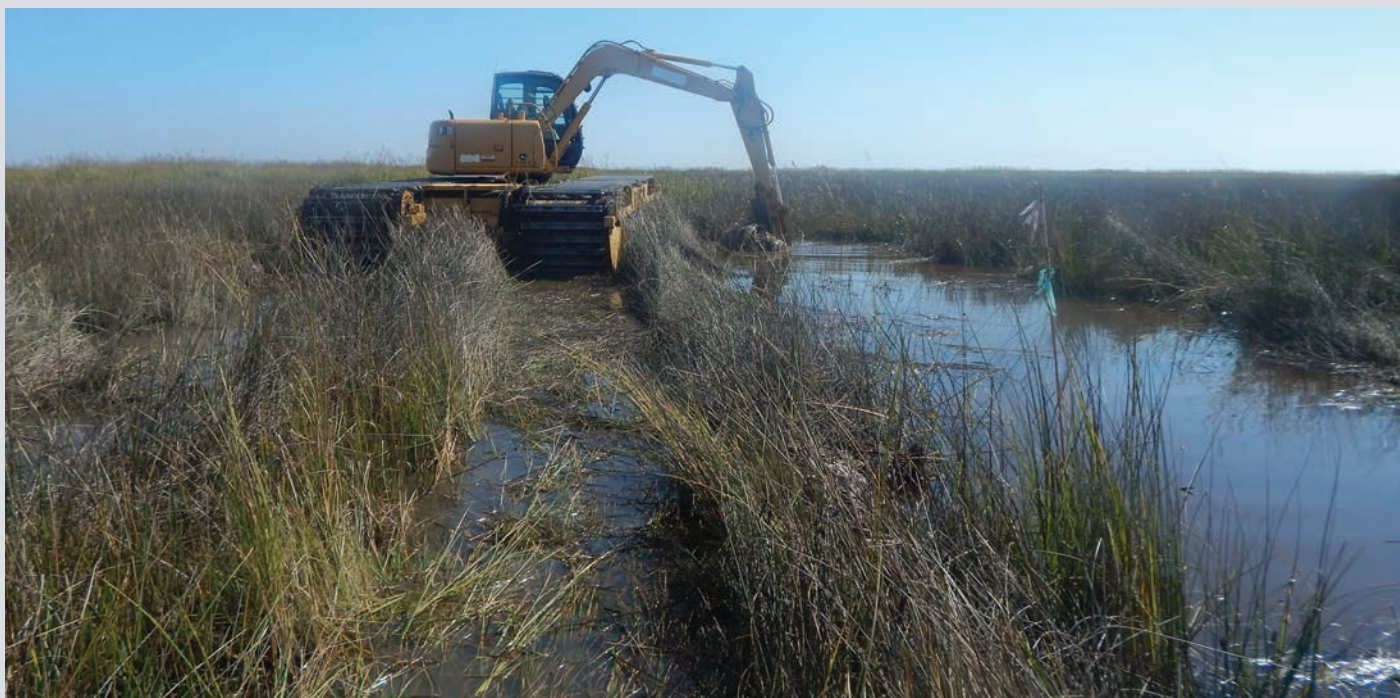
Audubon Maryland-DC has piloted the extension of tidal creeks into ponded areas to drain surface water and reinvigorate marsh vegetation at Farm Creek Marsh in Maryland. Dave Curson
