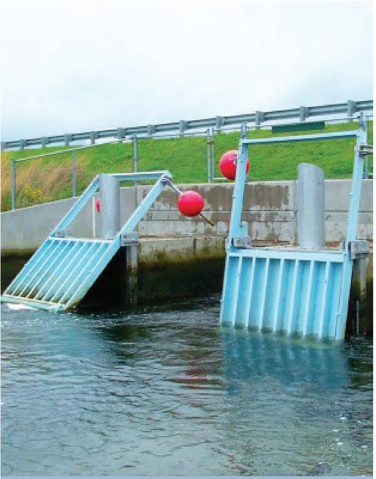
Self-regulating tide gates were installed during restoration efforts at Galilee Salt Marsh, Rhode Island. Waterman Valve LLC/ watermanusa.com
