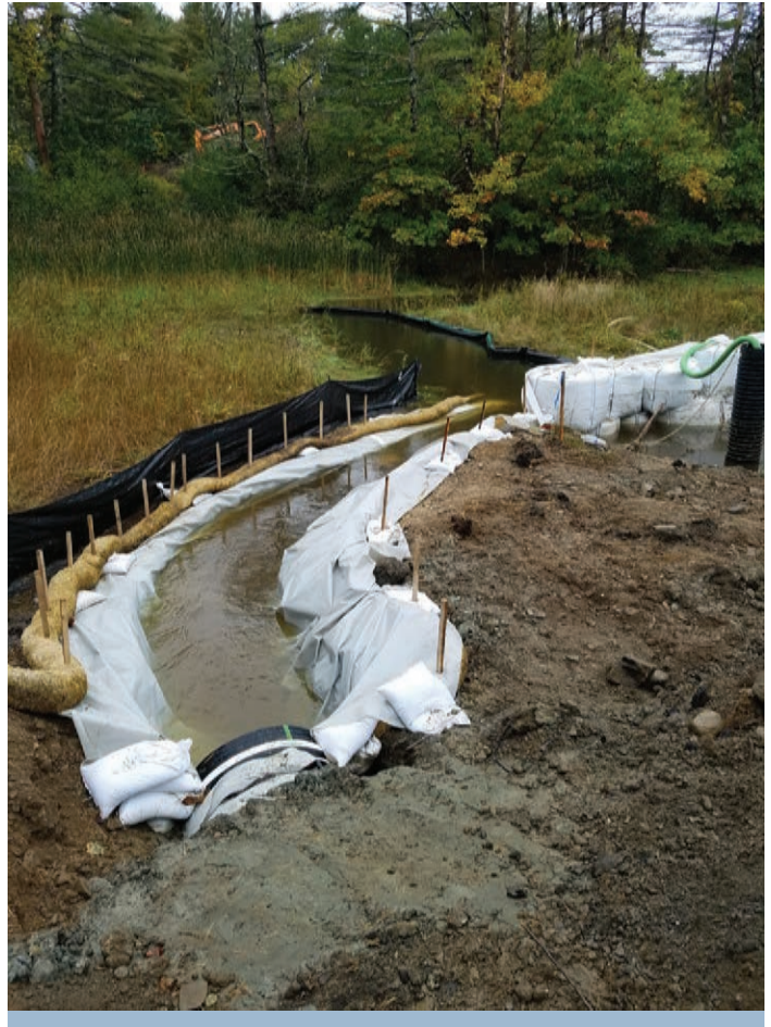
“Marsh smart” practices are those that support healthy tidal marsh structure and function such as replacing undersized culverts. Wells National Estuarine Research Reserve
