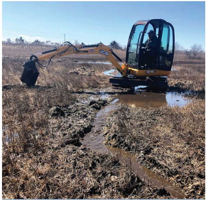
Placing peat on top of an existing marsh creates improved microhabitat conditions and may reduce flooding of Saltmarsh Sparrow nests. Wells National Estuarine Research Reserve
