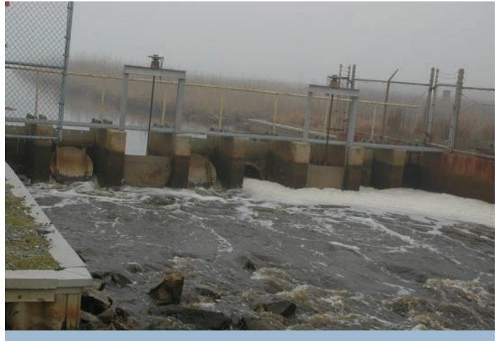
Water control structure from Prime Hook National Wildlife Refuge helps to manage flooding of saltmarsh habitat important for sparrows. USFWS
