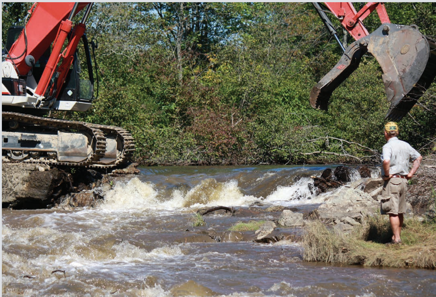
Rivers are a major source of sediment. Removing barriers like this one on the Goff Mill Brook in Maine allows sediment to flow into the Kennebunk River Estuary. The Wells Reserve
